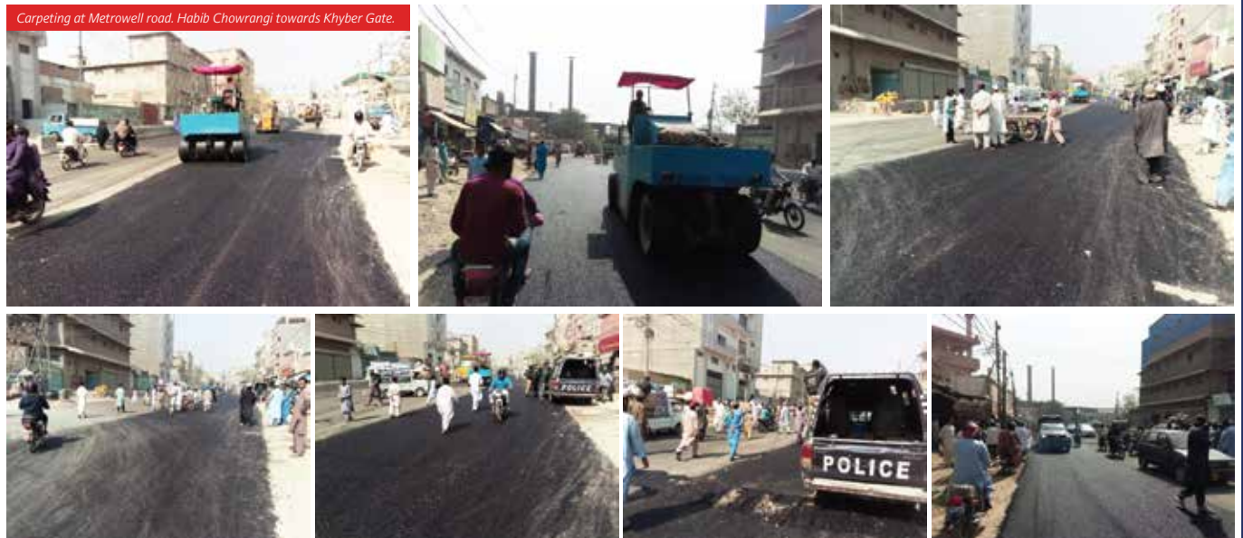
New road has been constructed from Jamia Binoria to GCT college.
